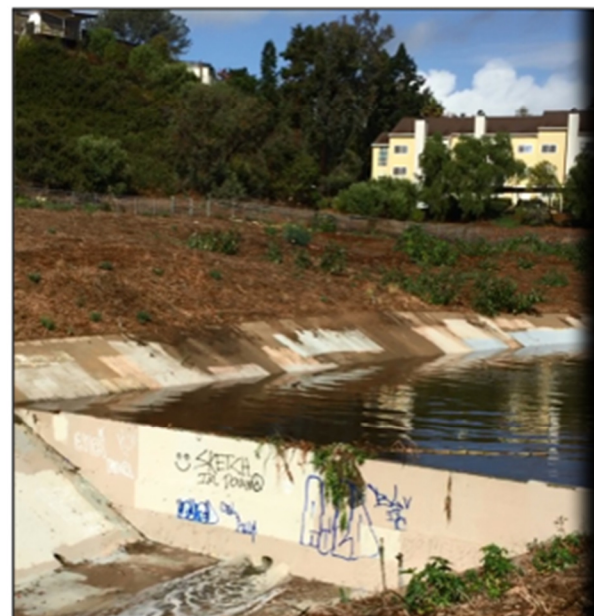
Stormwater sediment reduction basin (north view) after a storm event. The drainage channel discharges into the San Elijo Lagoon that is impaired by excessive sediment and bacteria.
