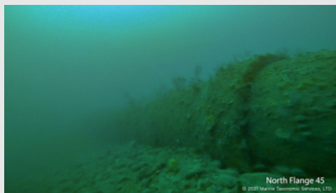
North Flange 45 © 2021 Marine Technology Services, LTD.
