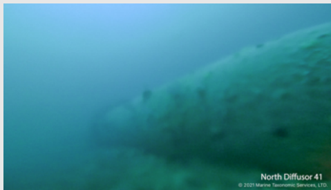
North Diffuser 41 © 2021 Marine Technology Services, LTD.
