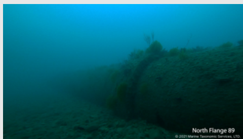
North Flange 89 © 2021 Marine Technology Services, LTD.
