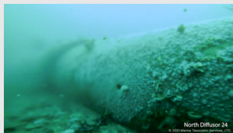
North Diffusor 24 © 2021 Marine Technology Services, LTD.
