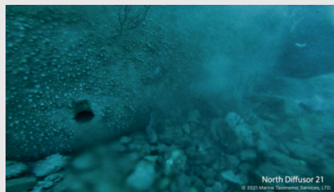
North Diffusor 21 © 2021 Marine Technology Services, LTD.
