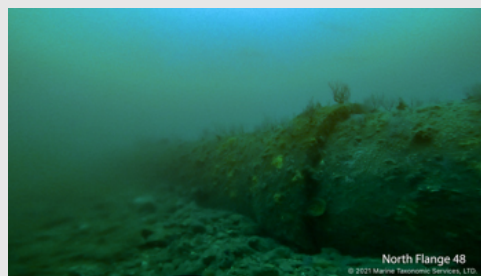
North Flange 48 © 2021 Marine Technology Services, LTD.
