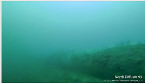
North Diffuser 93 © 2021 Marine Technomic Services, LTD.
