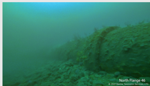
North Flange 46 © 2021 Marine Technology Services, LTD.
