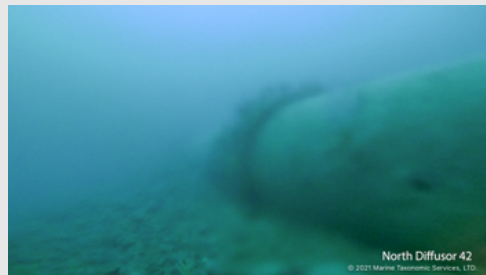
North Diffuser 42 © 2021 Marine Technology Services, LTD.
