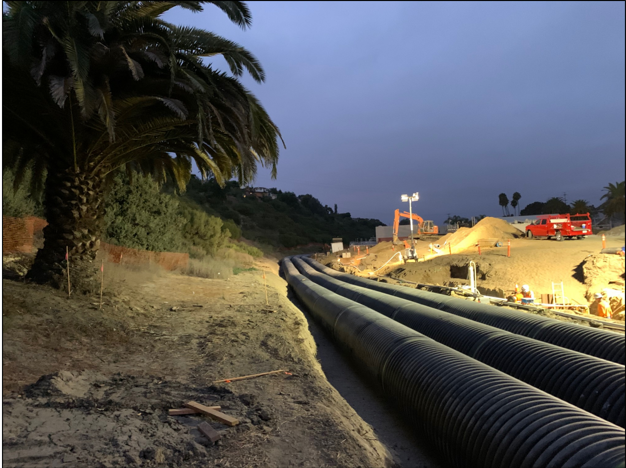
Figure 2. Contractor installed approximately 1,000 linear feet of three 5-foot diameter storm-drain pipes, which will be located under the new bike/pedestrian path.
