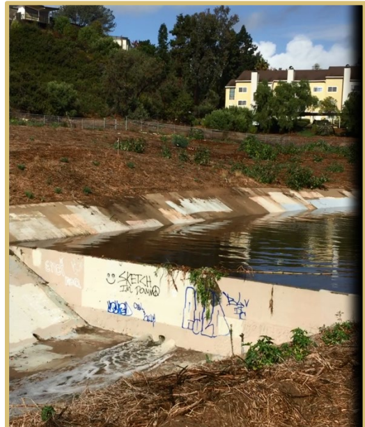
Figure 1 – Existing De-silting Basin
