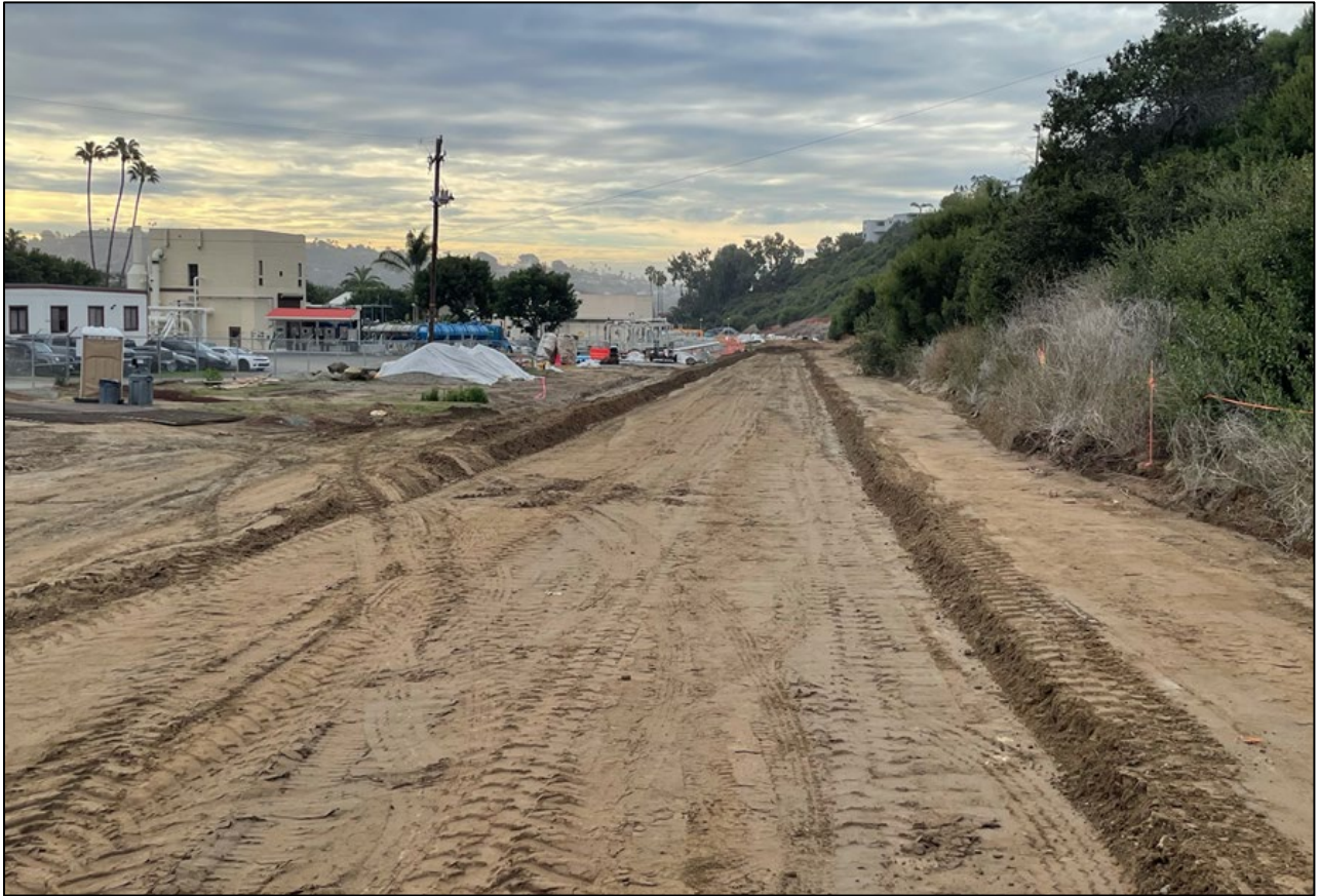
Figure 4. Multi-Use Path grading
