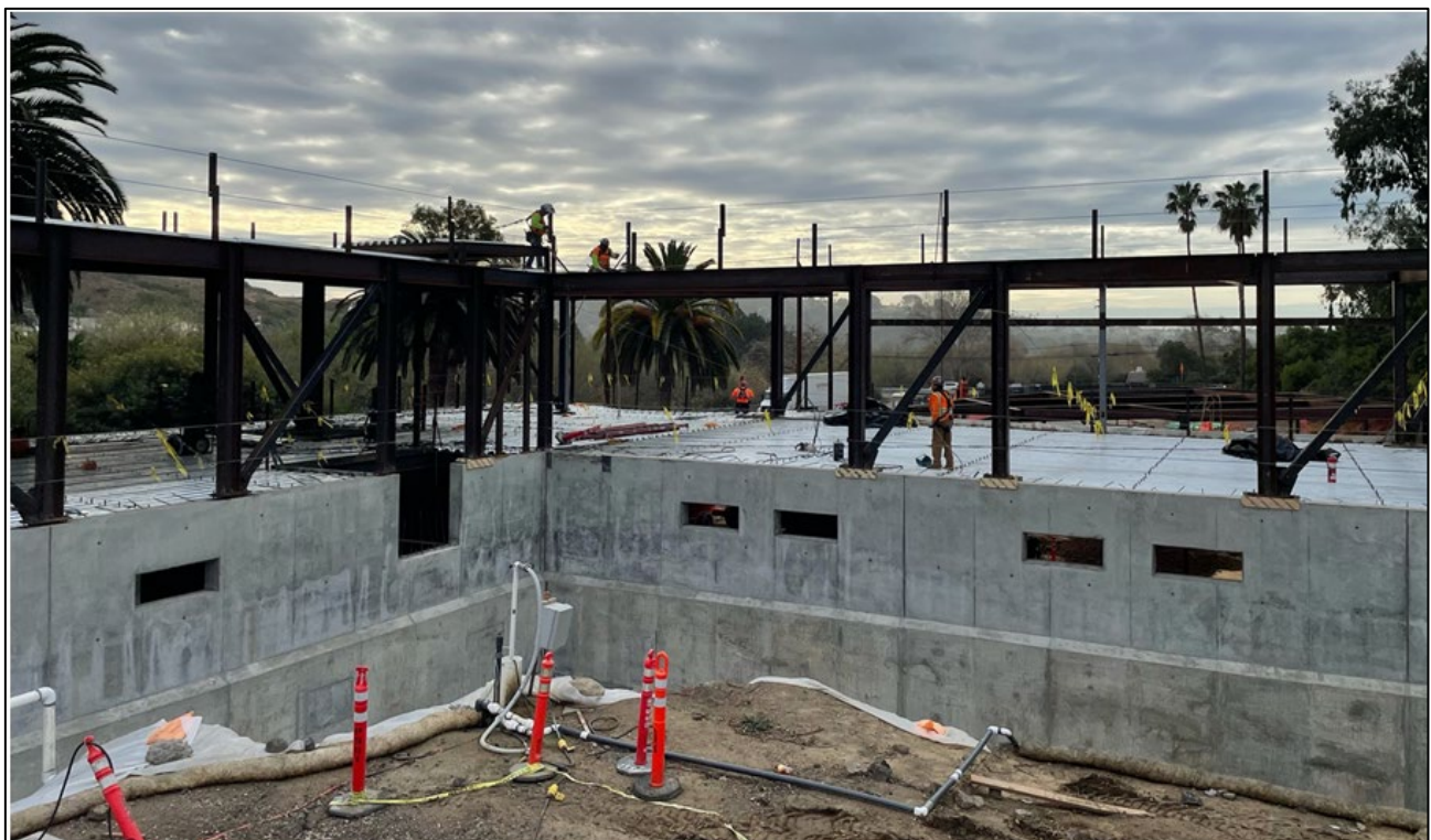
Figure 3. Building walls and structural steel framework
