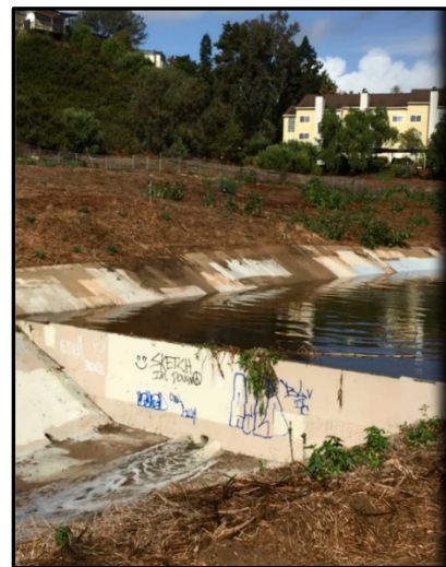
Figure 2 – Existing concrete storm channel and desiltation basin.
