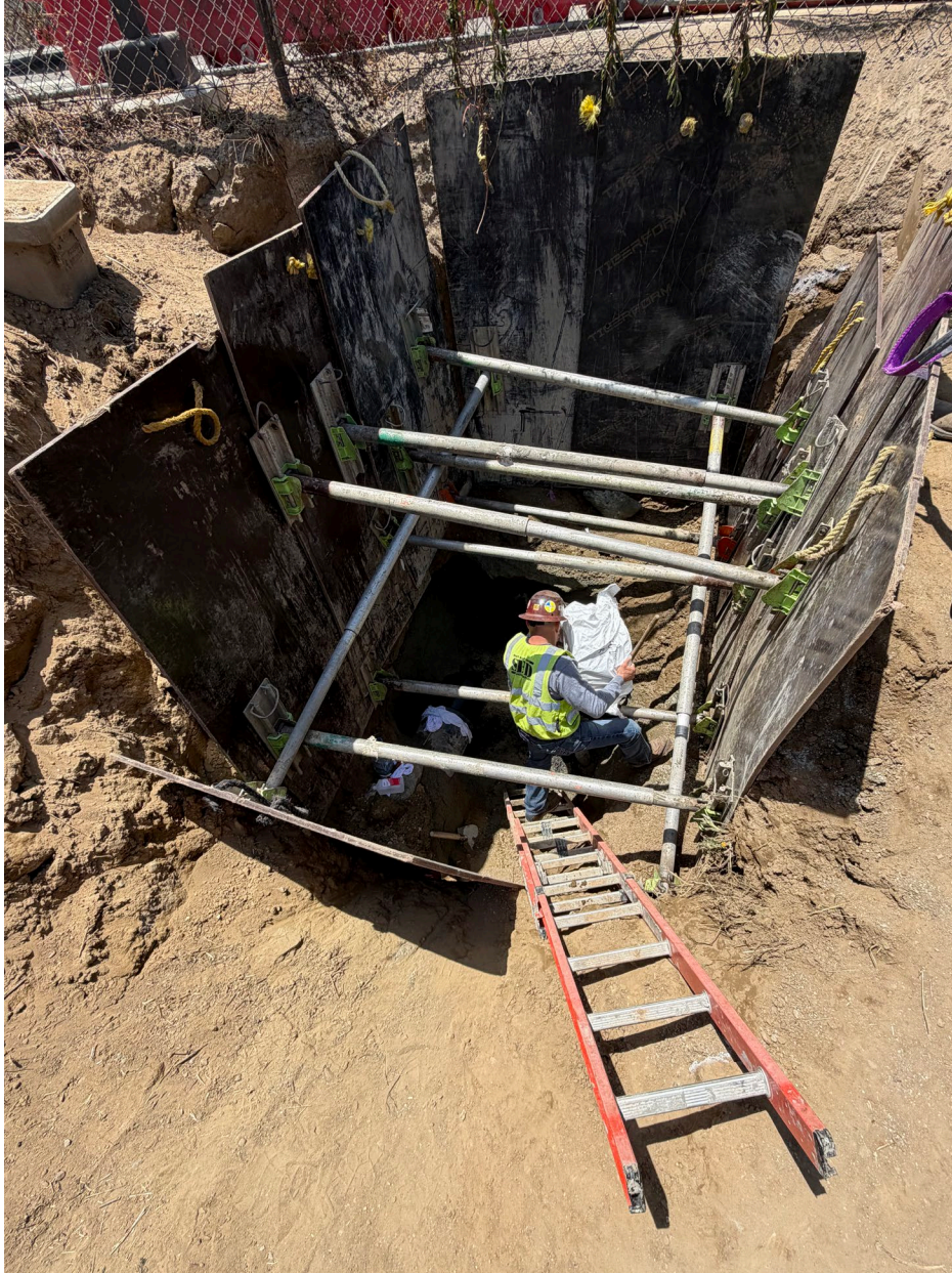
May 22, 2026 Pipe Repair In-Progress
