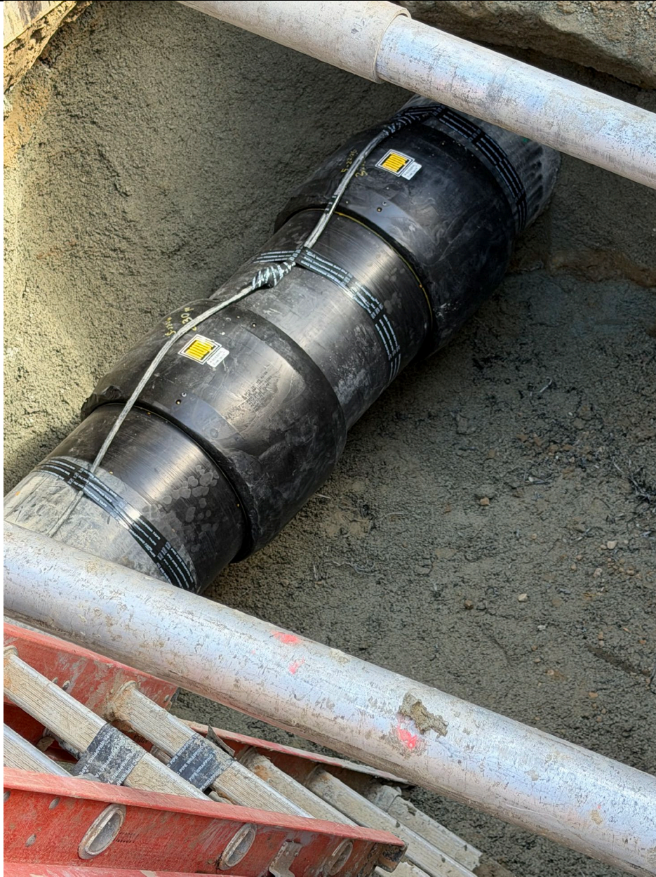
May 22, 2026 HPDE Electrofusion Couplings and Straight Pipe Replacement
