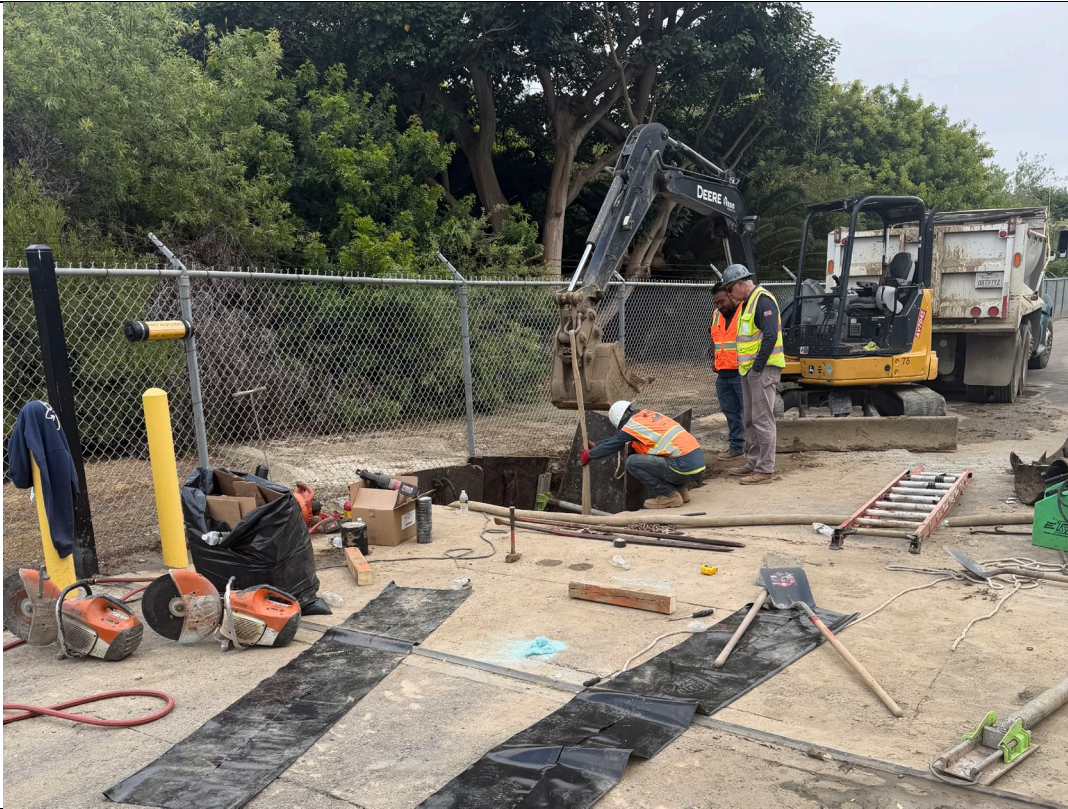
May 8, 2026 Pipe Repair In-Progress
