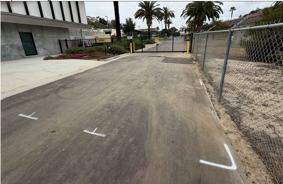
May 8, 2026 Excavation backfilled to grade with temporary asphalt Pavement repair area marked out with white paint
