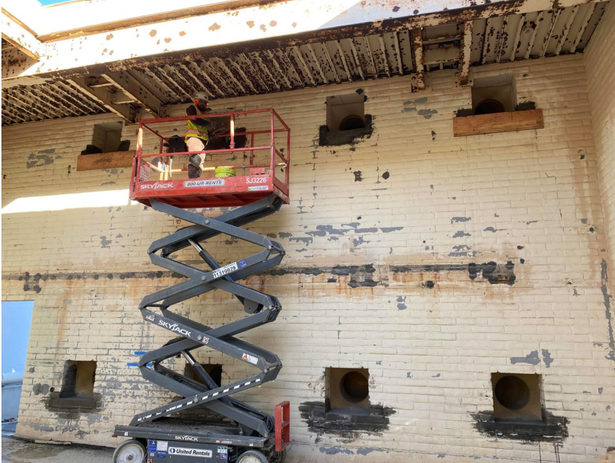
Photo 3 – Repairs in Progress (November 2024)
