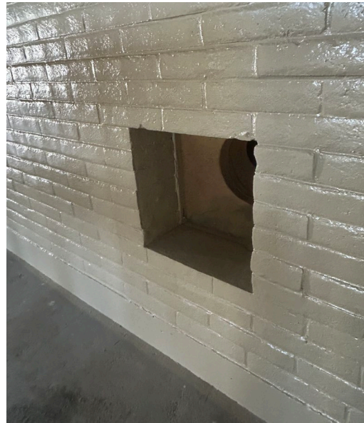
Photo 2 – Example of completed repairs
