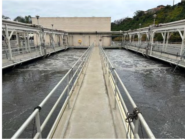
Continuous operation of the secondary process will be maintained throughout construction.
